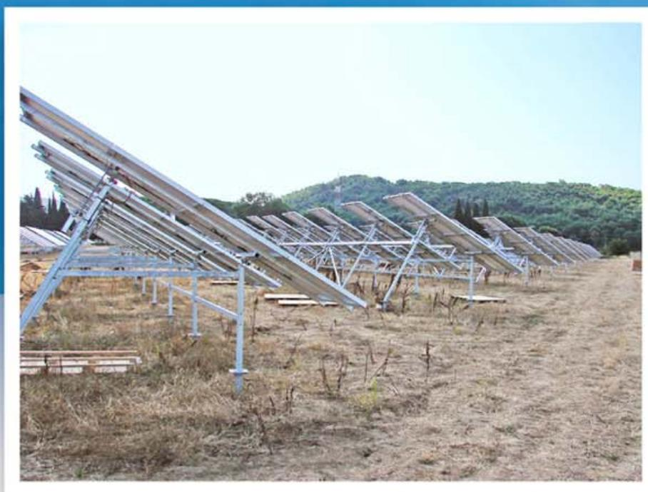
*The upper revolving support is considered a single-block, that acts as a support and fastening through thief-proof systems of the photovoltaic modules.*
