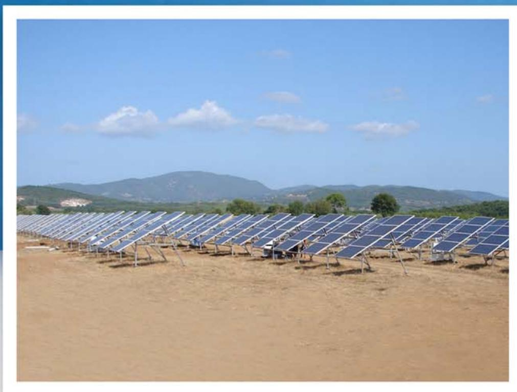
*The carrying structure is considered a single-block, that acts as a base and support to the superior frame for the assembly of photovoltaic modules.*
