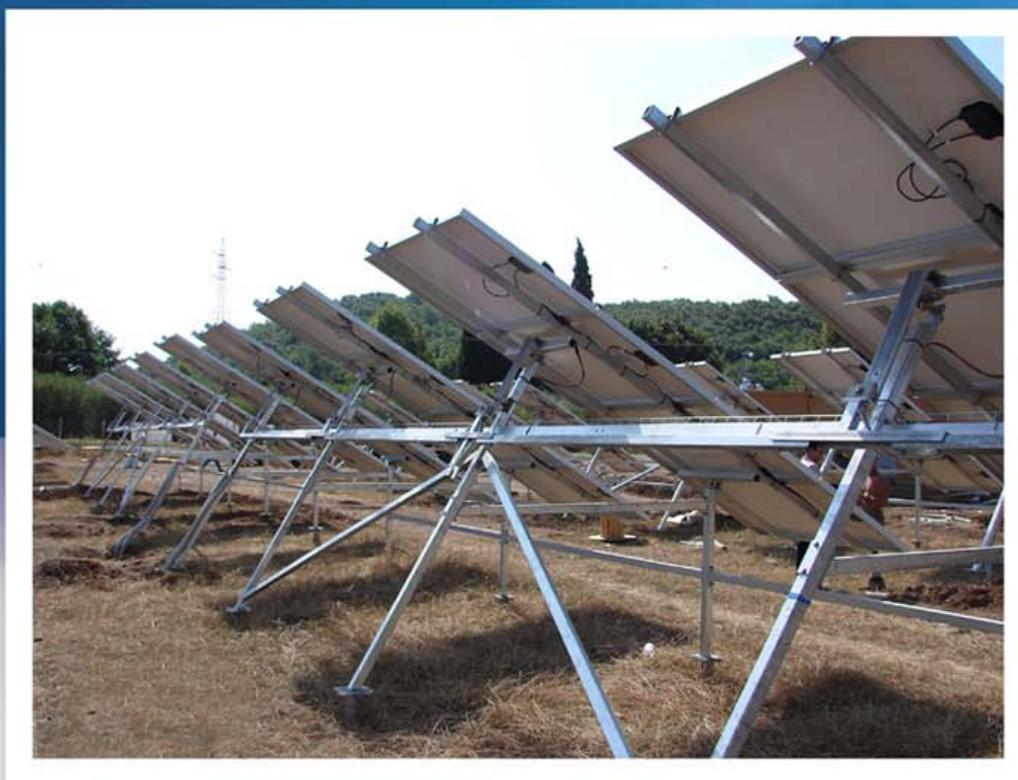
*In the mechanization of the system of movement, the thrust bars, connected to a system operated by an electric actuator, interact directly on the lever arms of the revolving supports for photovoltaic modules and allow their movement, according to the best program managed by software.*
