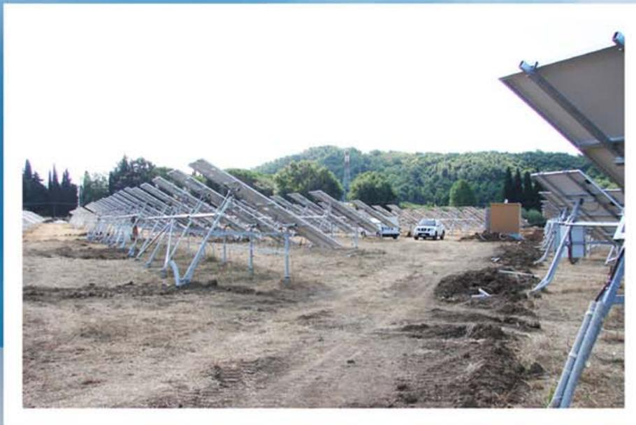
*This model of solar tracker works with the management of an astronomical program or, as alternative, with a rightness sensor program.*
